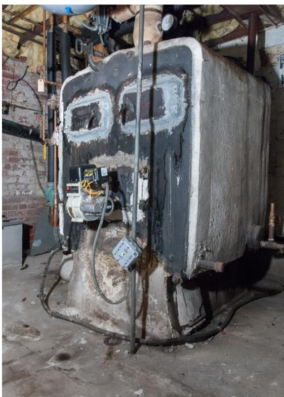
Basement boiler with asbestos blanket
